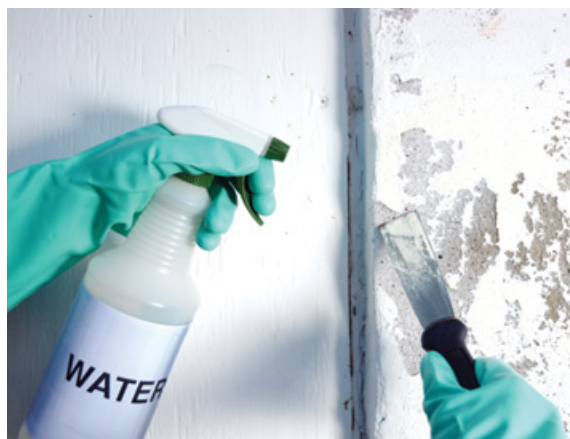
PHOTO: Wet-misting lead paint reduces dust hazard.
