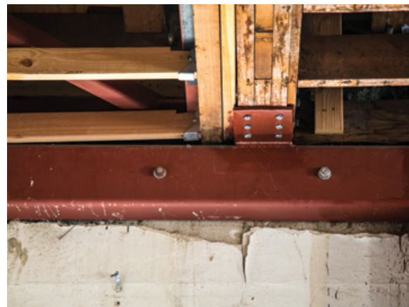
PHOTO: Steel structural support added for earthquake resistance.
